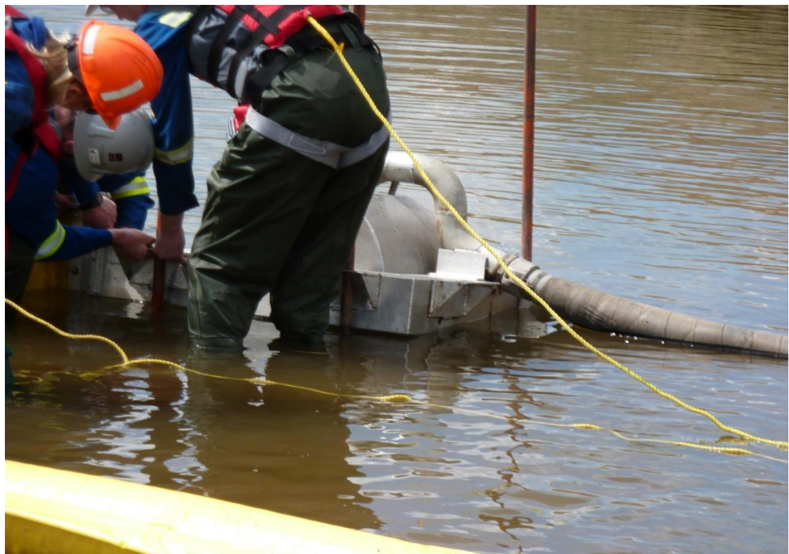
BOOM AND FLOATER HOSE BEING CONNECTED TO SKIMMER
